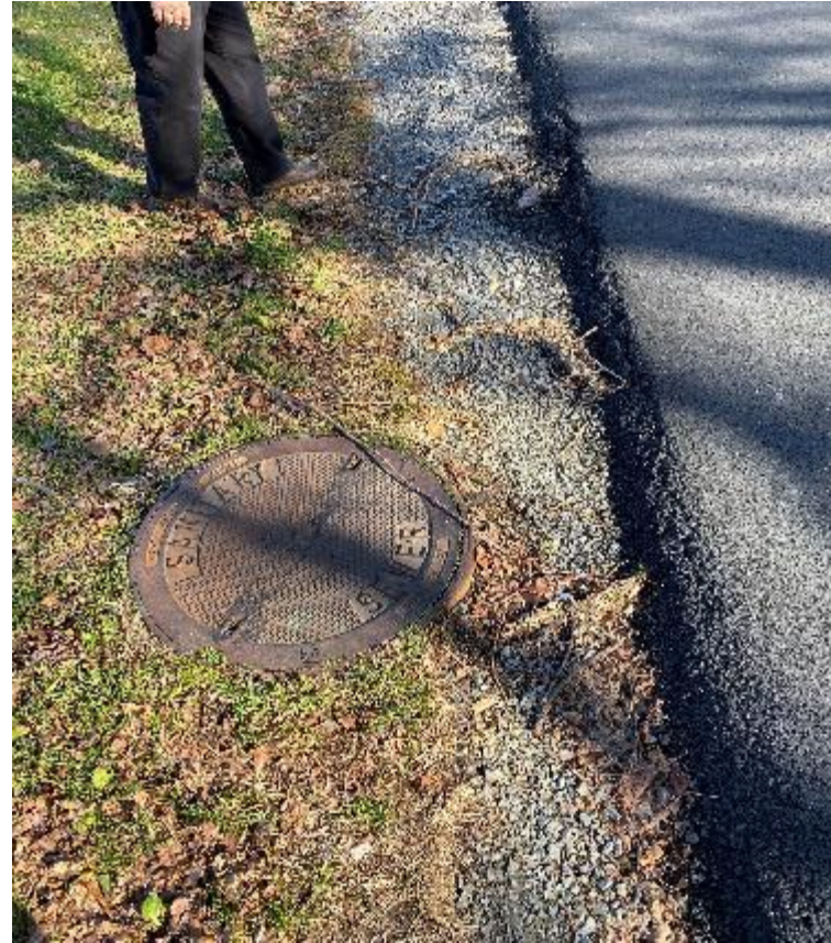
Existing utilities proximity to the roadway
